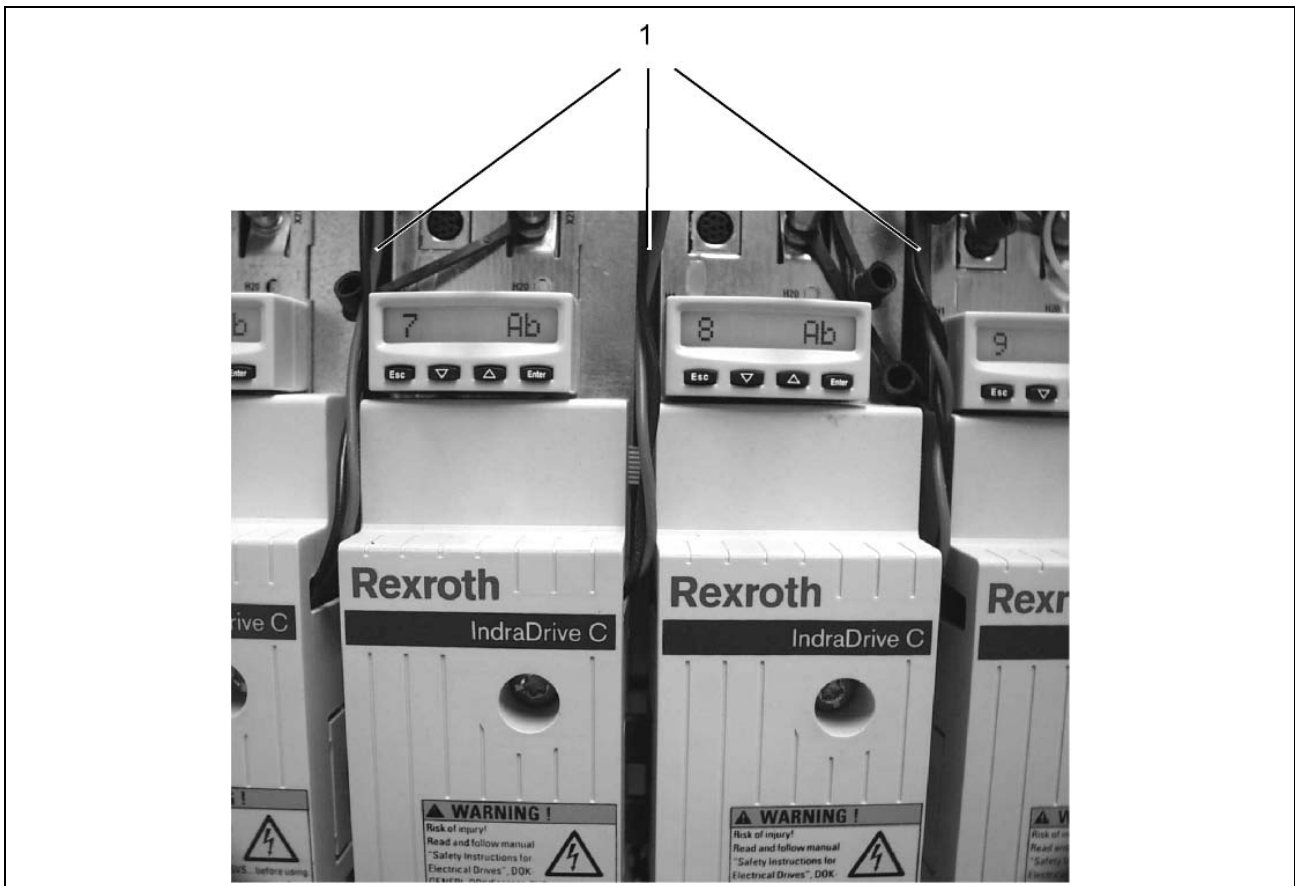
Fig. 6-77: Control voltage supply at X13
