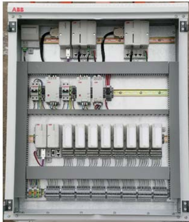
Figure 4. Cabinet with Controller and I/O on metal sheet
